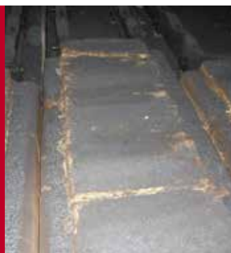
Photo 11 - Traditional Solution, cracks in blocks after 12 months.
