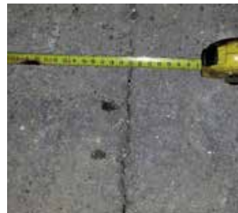
Photo 5 - Eredi Scabini Solution, joints in blocks after 12 months.
