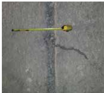
Photo 3 - Traditional Solution, joints between blocks after 12 months.
