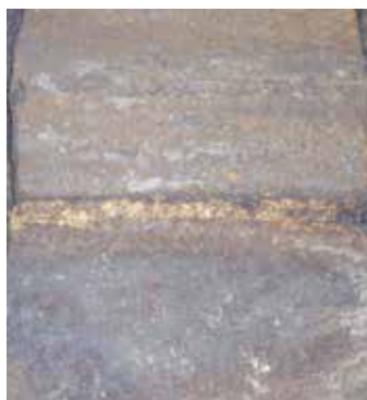
Photo 10 - Traditional Solution, joints between blocks after 12 months.
