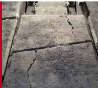
Photo 4 - Traditional Solution, cracks in blocks after 12 months.
